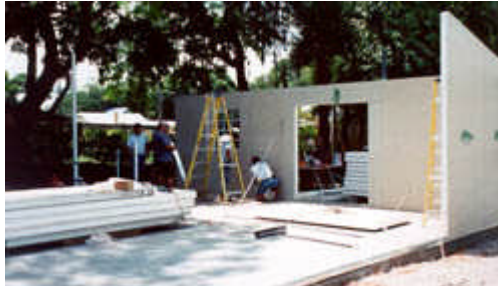
Wall erection process
