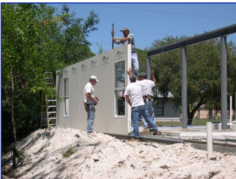
A four man crew can quickly and easily install the Home Front, Inc. SIP walls.
