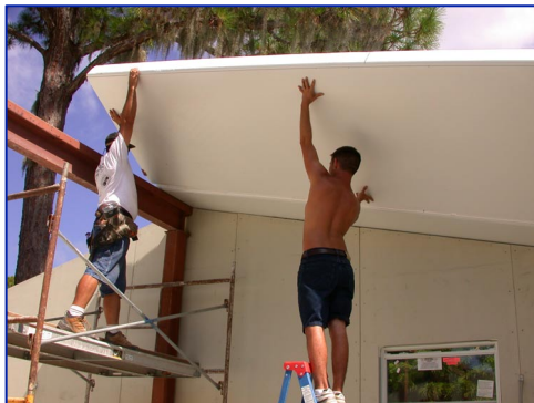
SIPs can also be installed as roofing or flooring systems.
