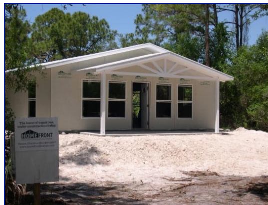
A Home Front, Inc. residence can be dried-in after about 3 days with a shell cost of approximately $35 per square foot.
